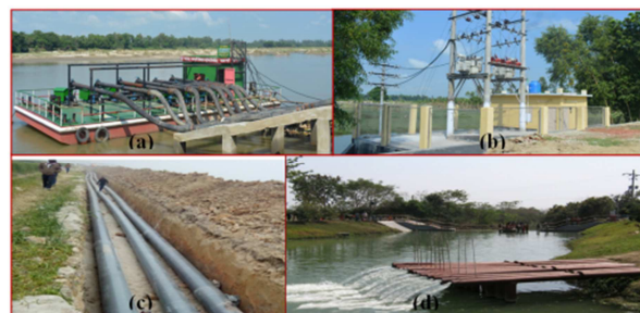
Figure 7. (a) Pontoon with centrifugal pumps and armed hose pipes, (b) Electric Sub-station (c) Underground pipe lines to carry river water to the canal, ponds or places to be irrigated, (d) discharging river water to the canal.
